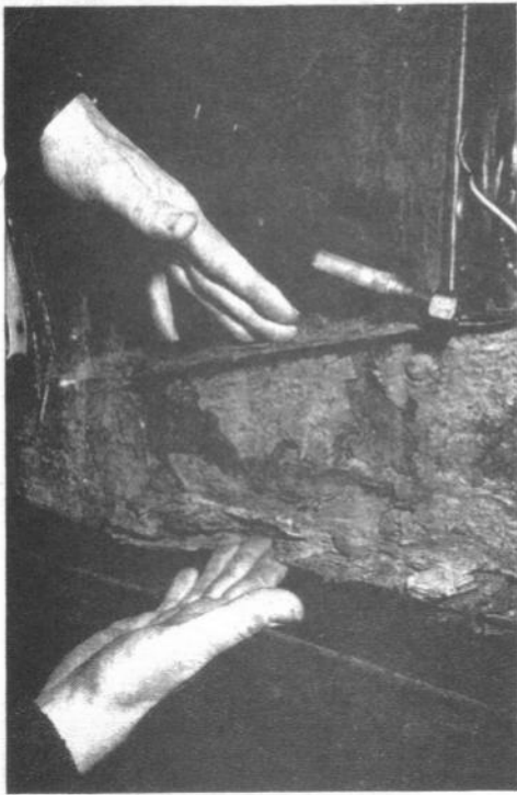
Inadequate rust protection means a rebuild almost always starts with a new chassis
